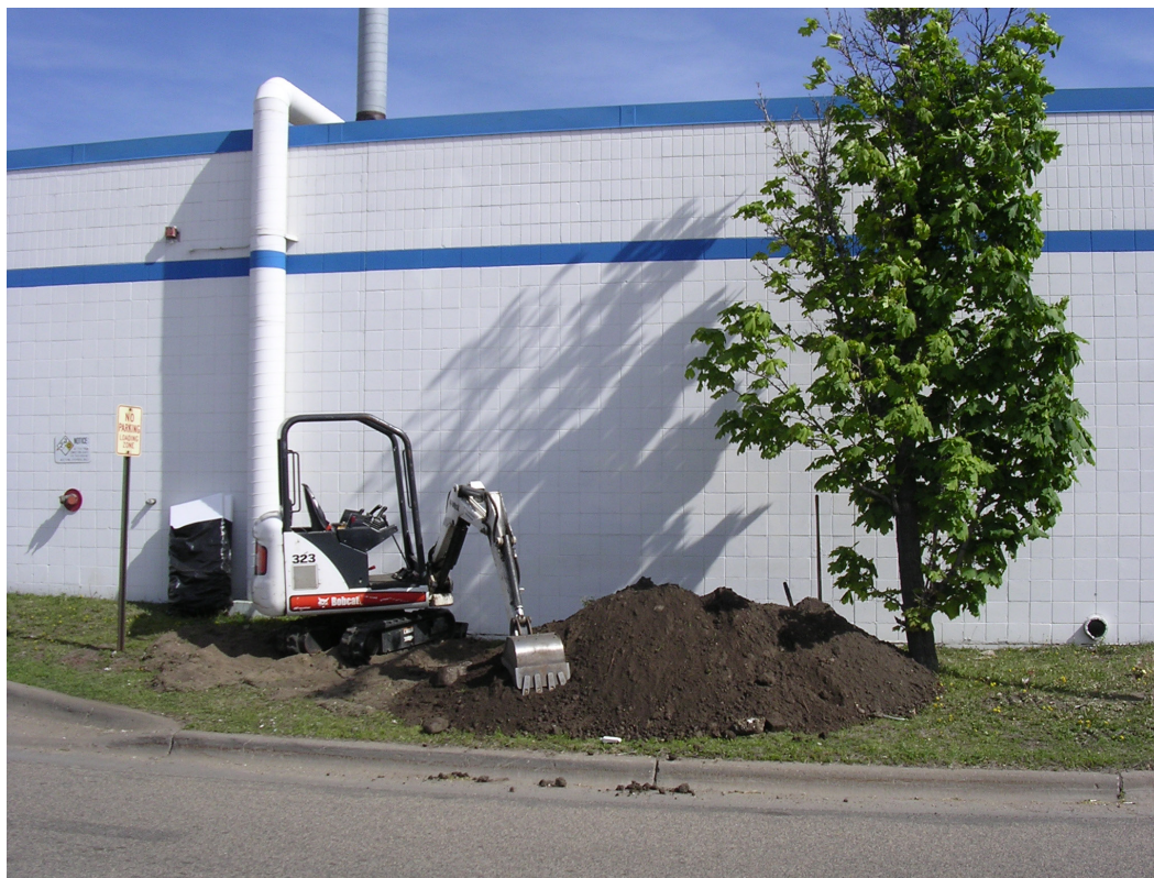
Figure 1. Excavation of insulation samples after 15 years
