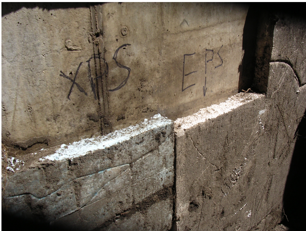
Figure 3. XPS and molded polystyrene were installed adjacent to each other
