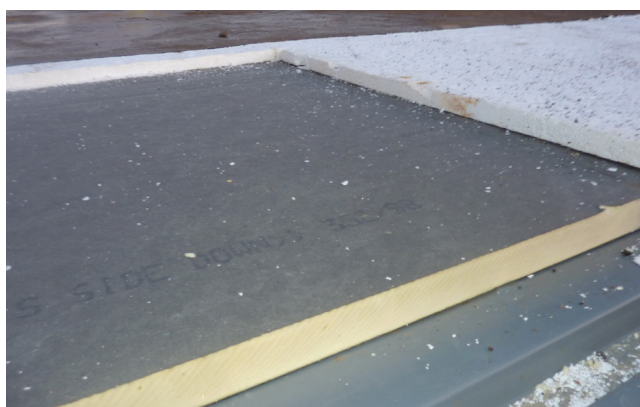
Figure 3. Existing roof being removed
