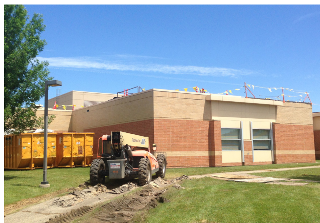
Figure 2. Roof replacement in progress
