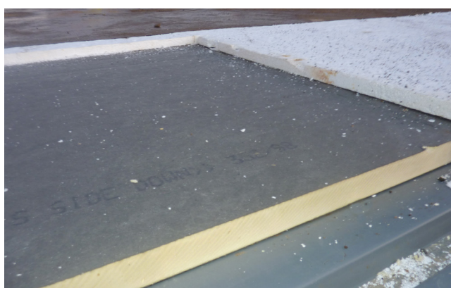
Figure 3. Existing roof being removed
